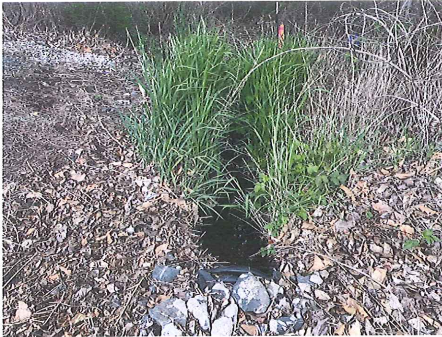
Photo 15. View north over culvert outlet and ditch draining to Wetland K (5/4/22).
